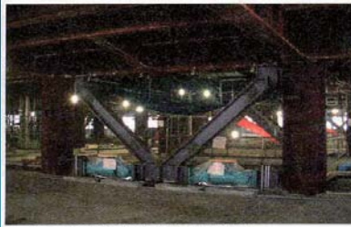
세미액티브오일댐퍼 (六本木ヒルズ森タワー) Semi-active Oil Damper (Roppongi Hills Mori Tower)
